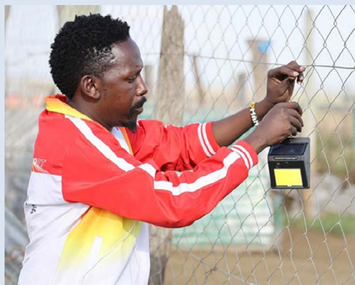
David Pesi installing lion deterrent light in one Boma at Enkikwei
