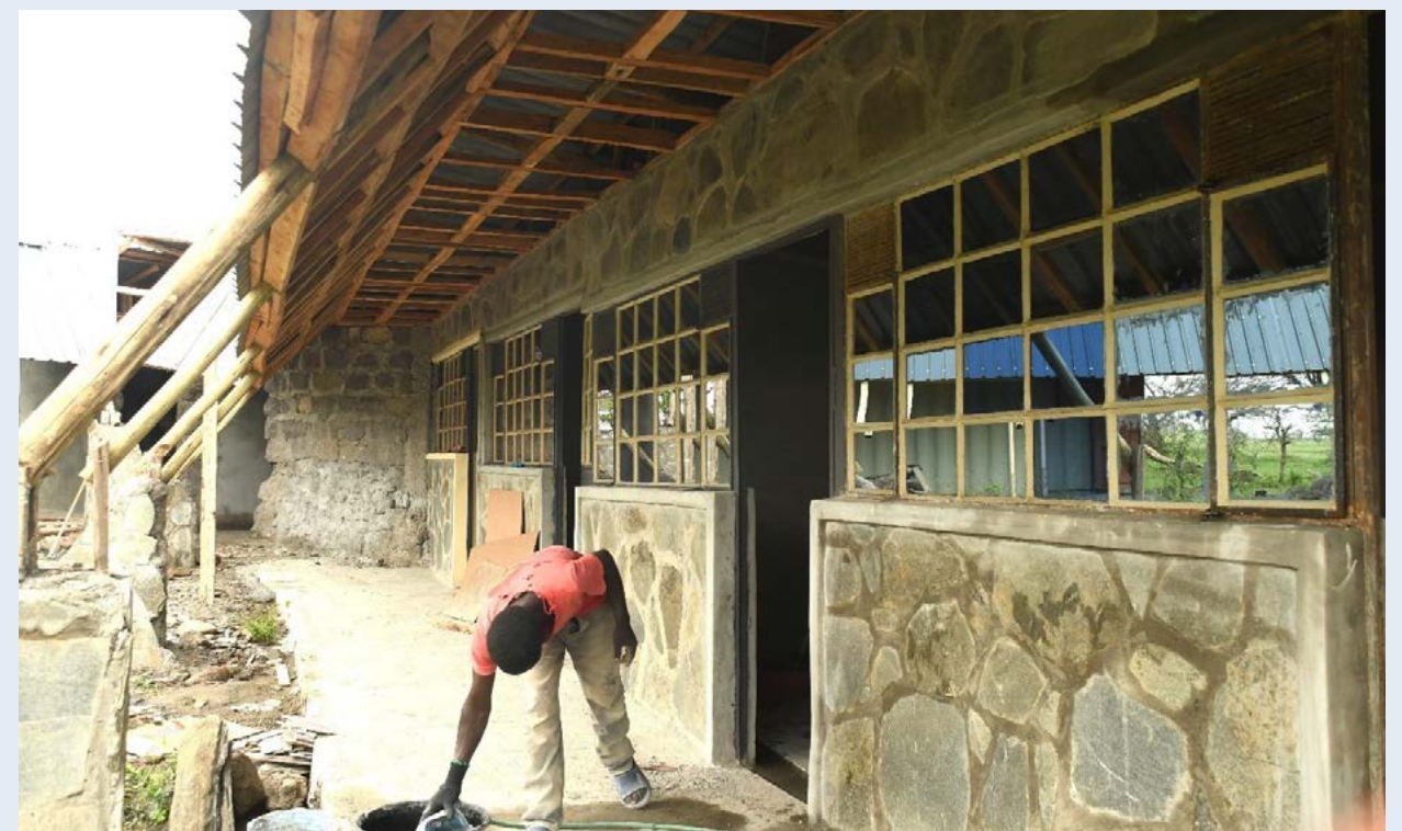
Staff accommodation ongoing construction
